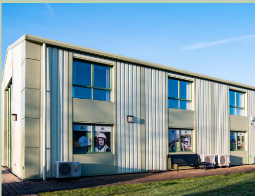
BSG SOUTH WEST TRAINING CENTRE, BRISTOL BSG South West Training Centre 5 Pinkers Court, Briarlands Office Park, Gloucester Road, Rudgeway, Bristol BS35 3QH T: 0300 304 9080
