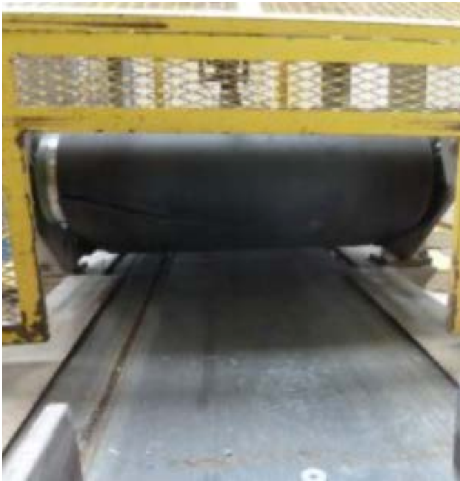
The bag flattening conveyor system. Image: Courtesy of HSE
